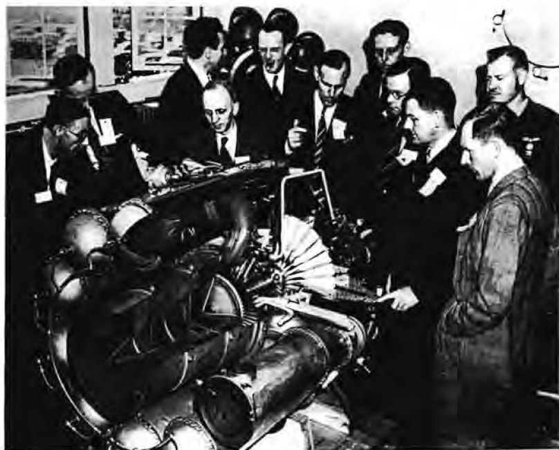
Above: Cutaway section of the I-A engine showing features such as the compressor, diffuser, air inlet guide vanes, combustor and turbine. Below: Donald F. “Truly” Warner (at center with glasses and cigar) hosts Frank Whittle (third from right) and the first British delegation to see the I-A engine, June 1942.
