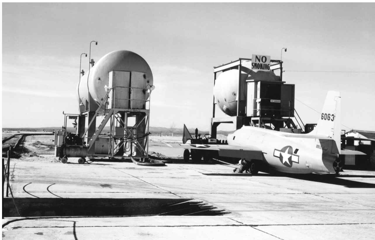
The No. 2 XS-1 on the ramp adjacent to the loading pit (lower left) and the lox and fuel loading facility, December 1946.
