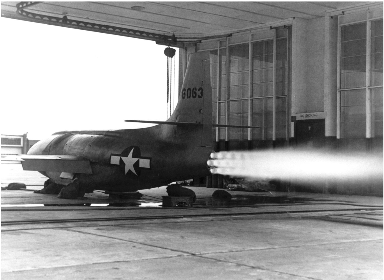
All four chambers of the XS-1’s XLR-11 engine ignited during ground tests in a hangar at the Bell plant in Niagara Falls, New York.
